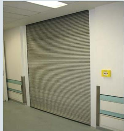
Effertz fire rolling door type "Fibreflam® Iso3" with a fabric curtain, classification EI30-C5 according to EN 13501-2 and EN 16034. Durability of mechanical performance approved for 200.000 cycles. Meeting the applicable safety requirements of the European door product standard EN 13241.
