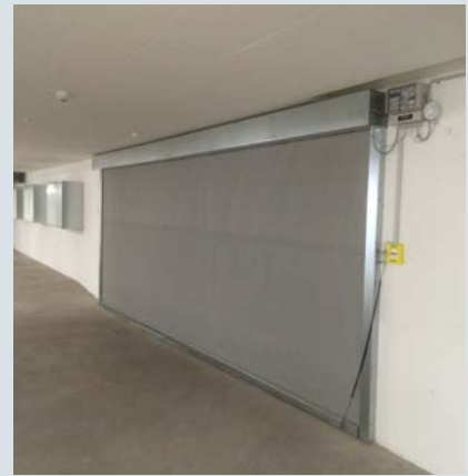
Underground car park
